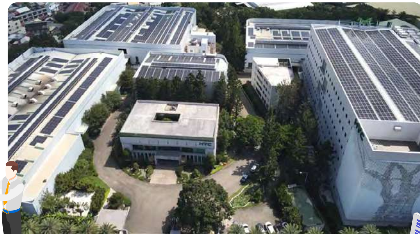
Caption | HYC factory-wide solar panel installation with a total installed capacity of 1,900 kWp
