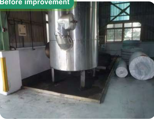
Caption | Before improvement: no protective barrier installed in heat medium tank area
