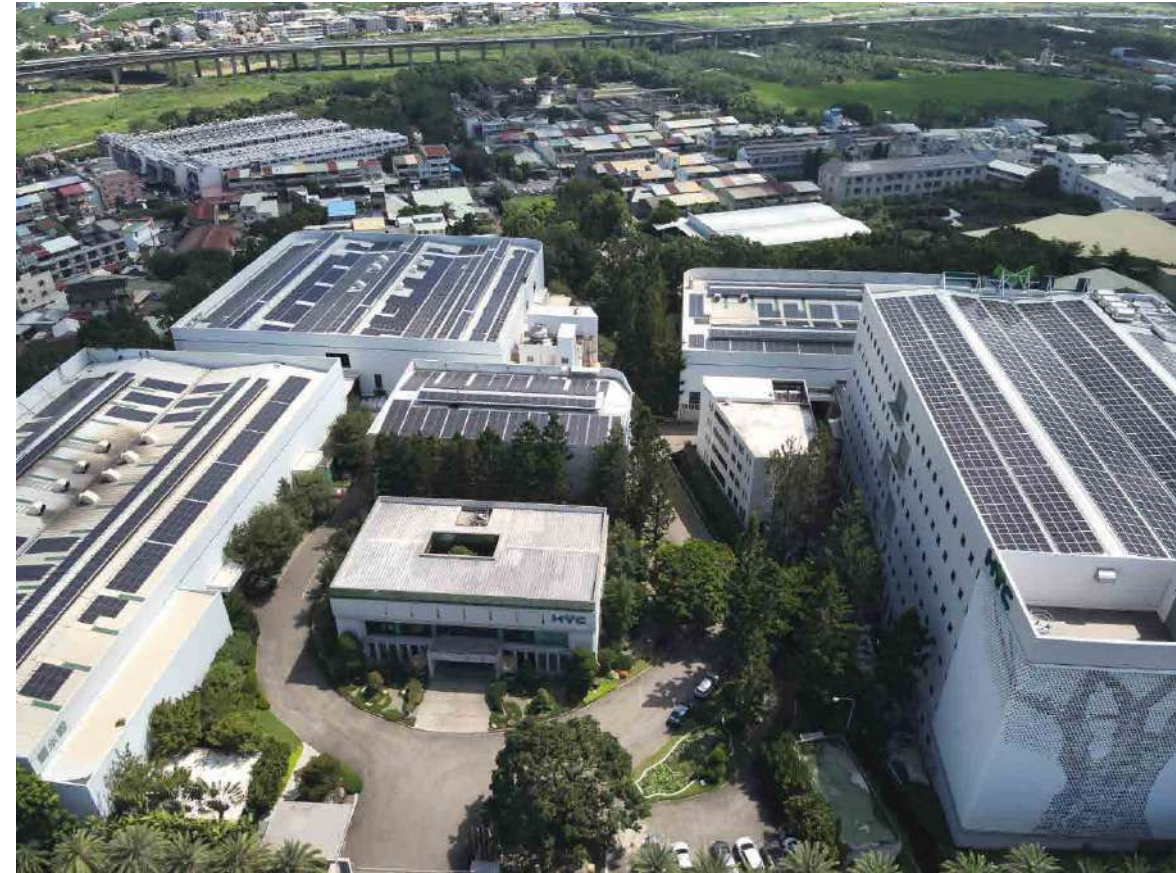
Caption : Solar Panels Installed on All Plant Rooftops, with a total installed capacity of 1,900 kWp
